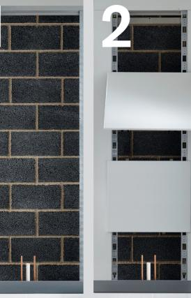
**02** Click-fix the first Frameduct unit onto the frame and slide into position. Open the mid panel to a fully hinged position. Attach a vertical flashgap to the frame on either side of the unit, screw-fixing to the frame from the face. Fix tie back to the wall. Repeat until all units are in place.
